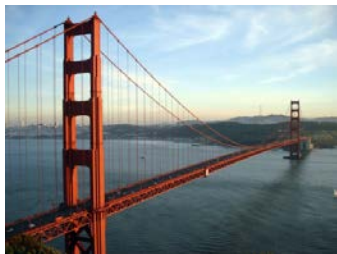
Golden Gate Bridge
